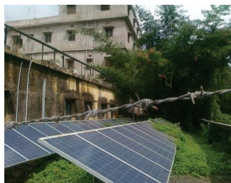
*(Solar plates of off-grid Solar Power Plant at Jasidih, Deoghar covered with grass)*
